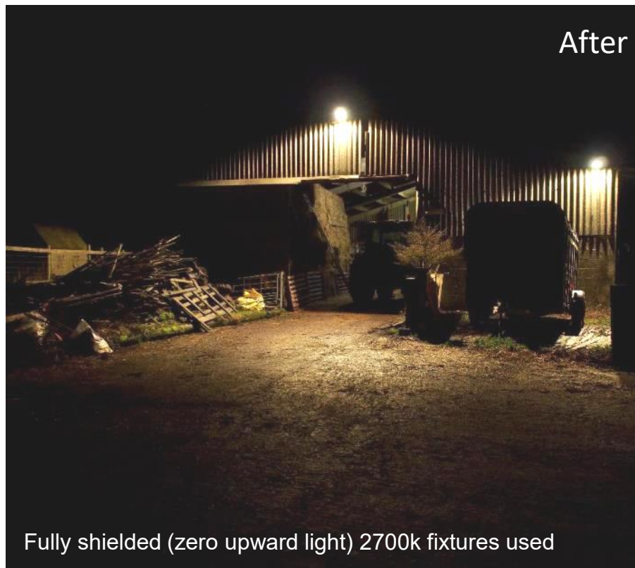
Low level driveway lighting instead of unshielded floodlights
