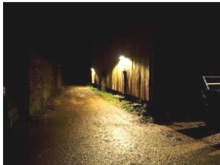
Low level driveway lighting instead of unshielded floodlights
